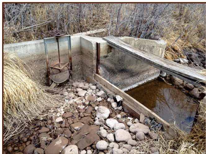
A lateral and structure of the UIIP Uintah Canal in poor condition.
