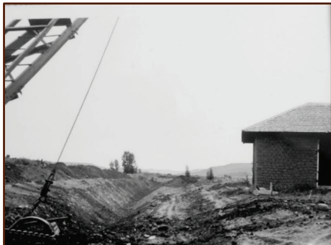
Rehabilitation of a Tribal canal in the Pine River valley using a dragline – circa 1964.
