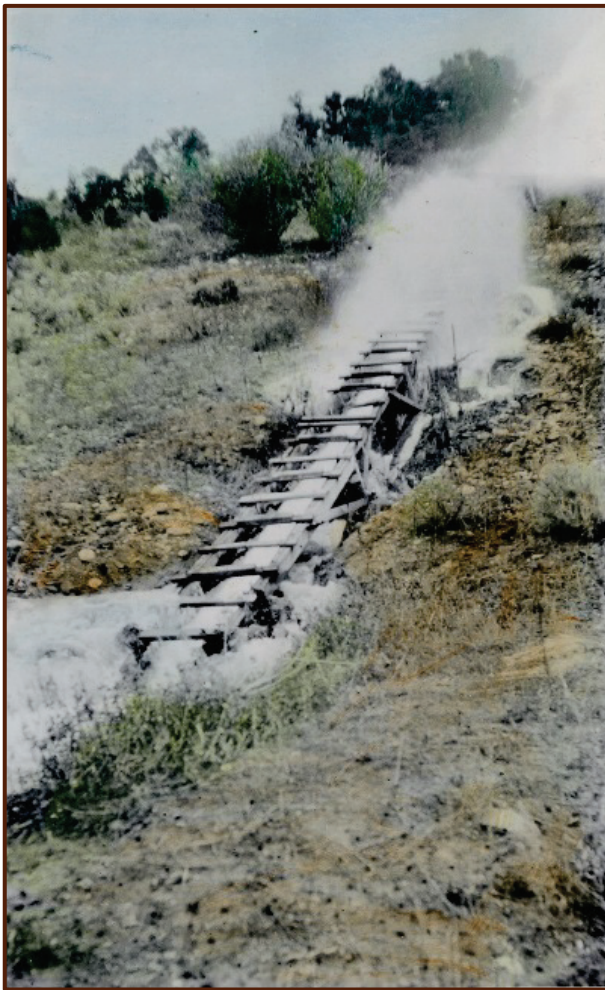
The broken terrain of the Southern Ute Reservation requires extensive engineering to convey irrigation water. A series of large drop structures on the Dr. Morrison Canal as it appeared in 1927 (above), and its modern configuration upon completion in 1959 (right).
