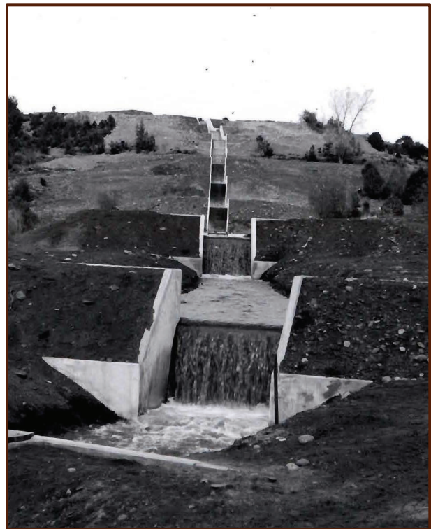
The broken terrain of the Southern Ute Reservation requires extensive engineering to convey irrigation water. A series of large drop structures on the Dr. Morrison Canal as it appeared in 1927 (above), and its modern configuration upon completion in 1959 (right).
