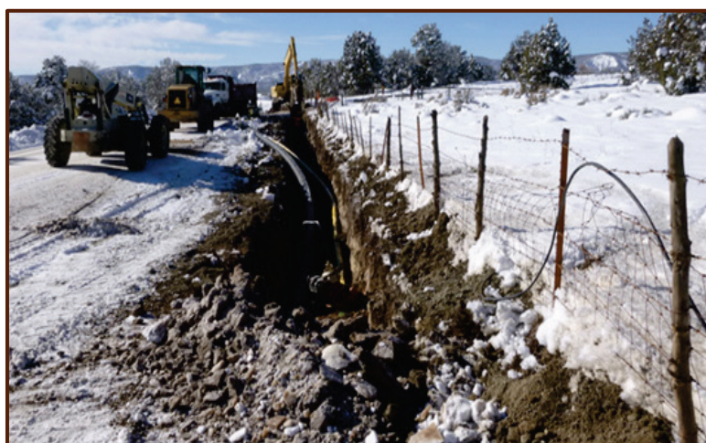
Rural domestic water systems can require miles of pipeline to serve only a small number of residences, increasing the per user costs for both construction and maintenance.
